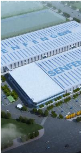
New headquarters (High-tech Zone, Jinan City)
